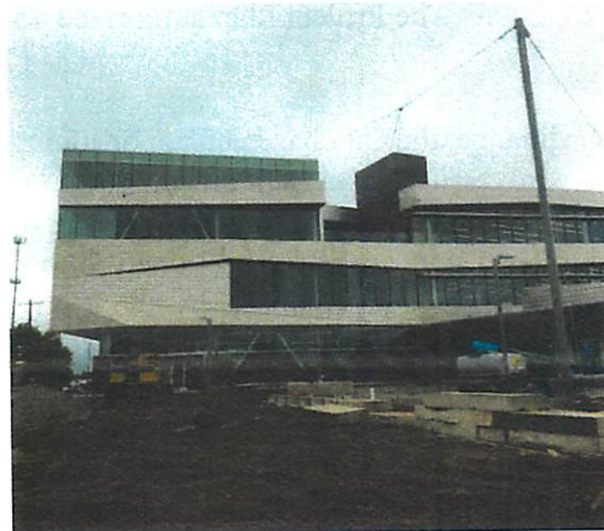
Norman Public Library, Central Branch (Under Construction)
